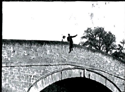
They meet where the bridge is
